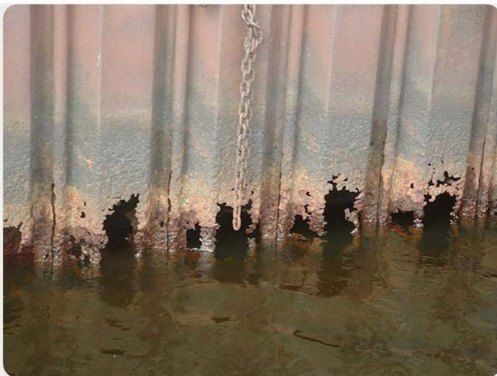
MIC of pilings in the Duluth Superior Harbor in Duluth, Minnesota. Photo courtesy of Gene Clark, University of Wisconsin Sea Grant Institute.
