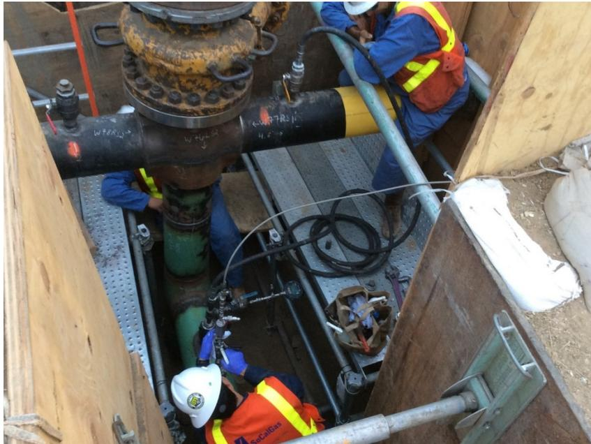
Any customers who were being fed by Compressed Natural Gas (CNG) or Liquefied Natural Gas (LNG) have their service switched to being fed from the new pipeline. The process for abandonment of the original line also needs to take place. It begins by purging, isolating ends and taps, and permanently decommissioning the line which typically takes a few days to complete.
