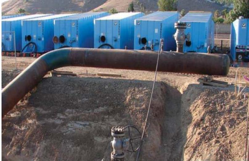
Filtration equipment is used to remove organic and inorganic material to permitted disposal levels. The water may be disposed of at a sewer, transported to a disposal facility via a truck, or provided to a third party for non-potable reuse. Permit requirements typically dictate how used hydrotest water is disposed.
