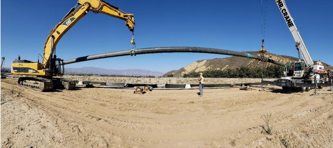
Figure 15: HDD Pullback
