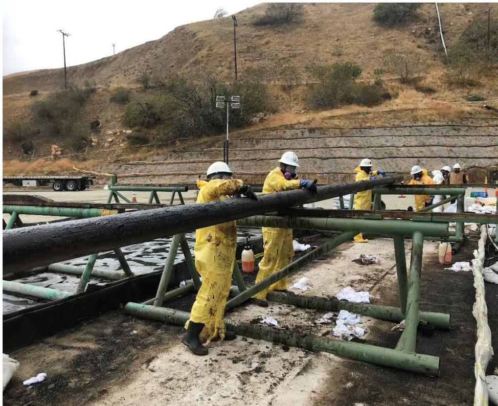
Figure 28: Cleaning a Joint of 7 in. Casing at PS-20
