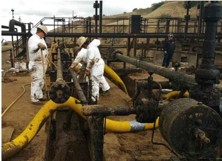
Figure 24: Cleaning of Pipe Trenches Using Supersucker® Vacuum Loader
