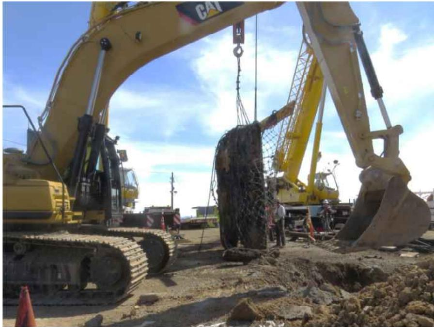
**Figure 13: Concrete Slab Removed from Crater by Crane**
