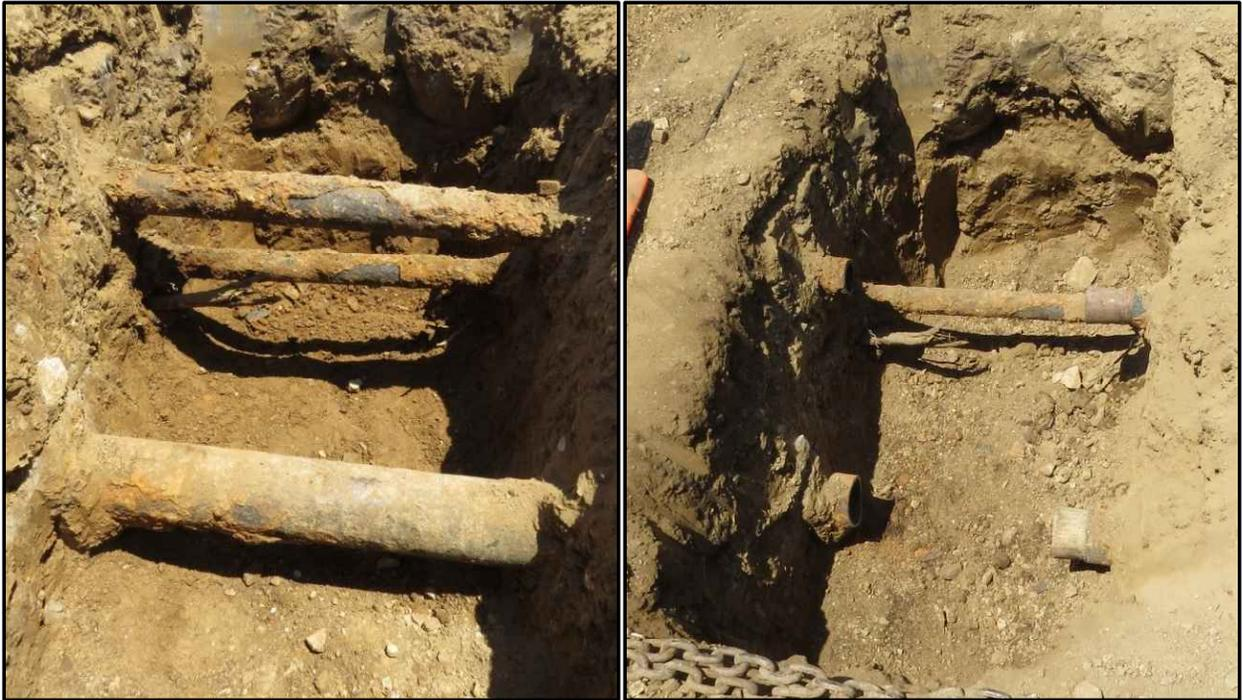
**Figure 30: Exposed Abandoned and Buried Flow Lines Uncut (Left), Cut and Plugged (Right)**
