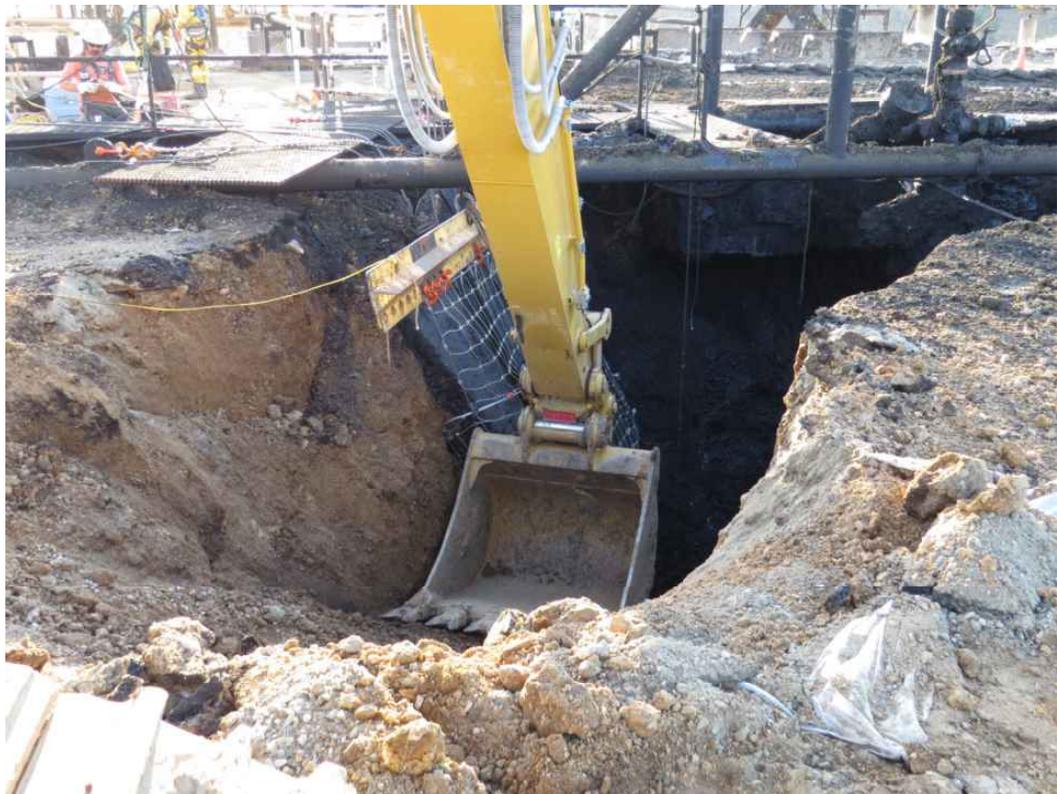
**Figure 10: Trench Excavated in Crater South Wall for Slab Removal**
