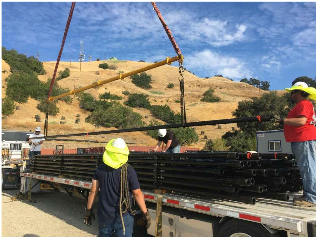
**Figure 20: Loading Tubing onto Bolsters at PS-20**
