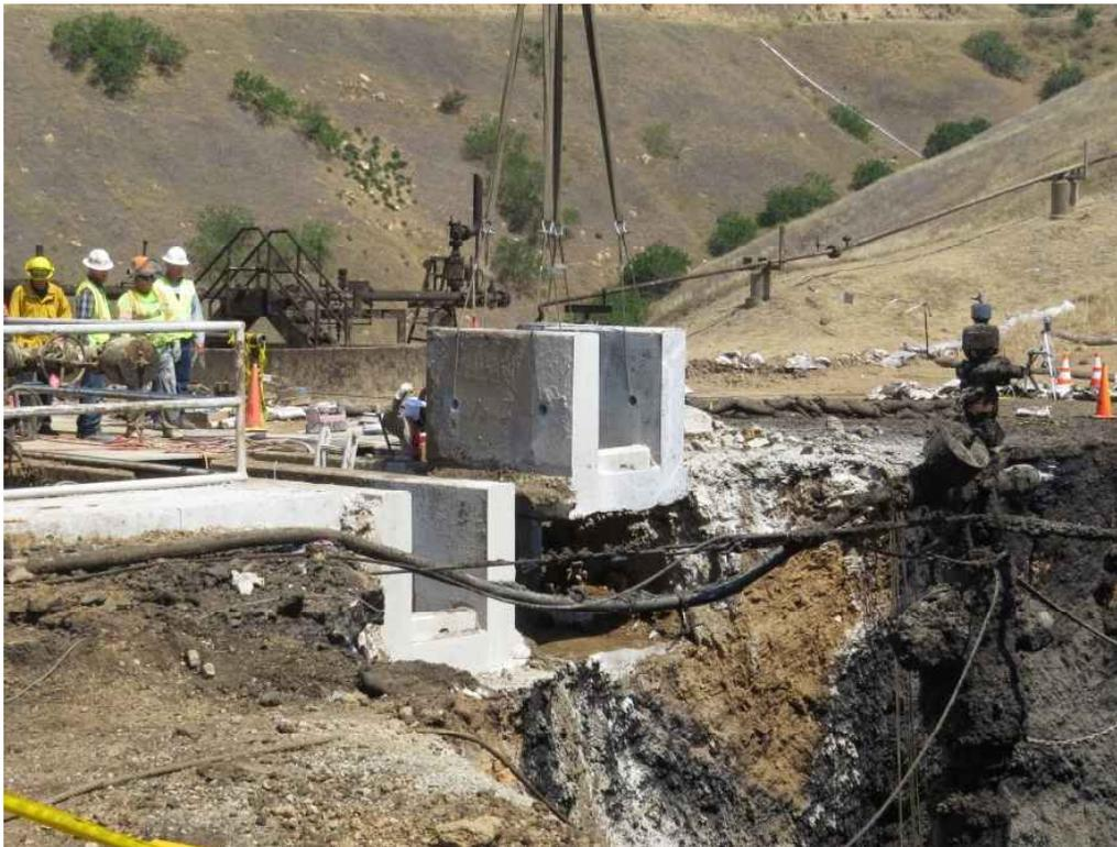
**Figure 28: Another SS-25 Pipe Trench Segment Removed with Crane**
