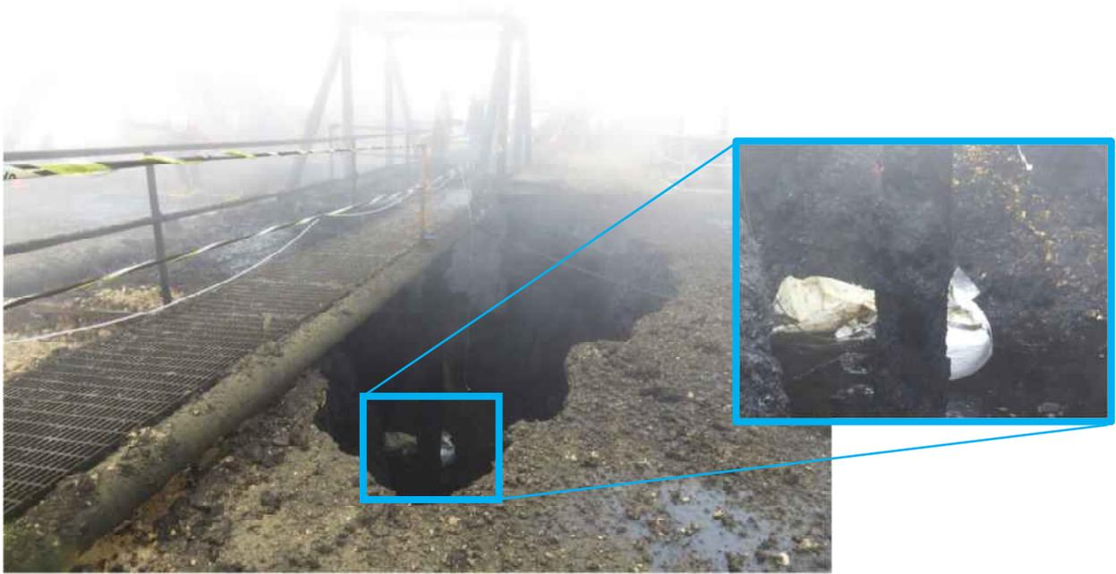
Figure 4: Placement of the First Super Sack Container
