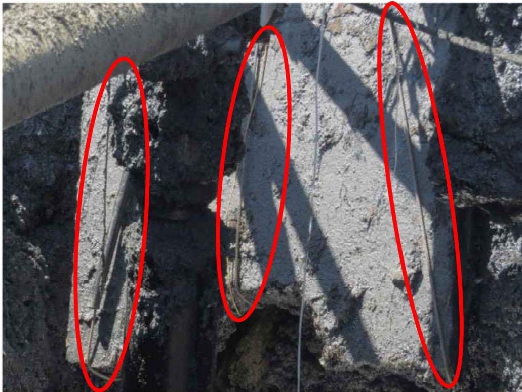
**Figure 8: Three Safety Straps Were Tightened around Slab**
