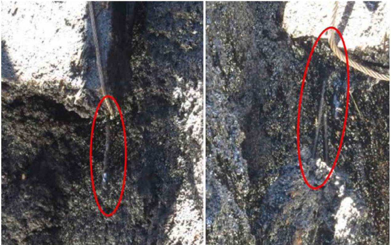
Figure 3: Visual Indications of Rebar
