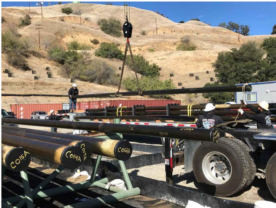
Figure 36: Loading the 7 in. Casing onto Bolsters at PS-20
