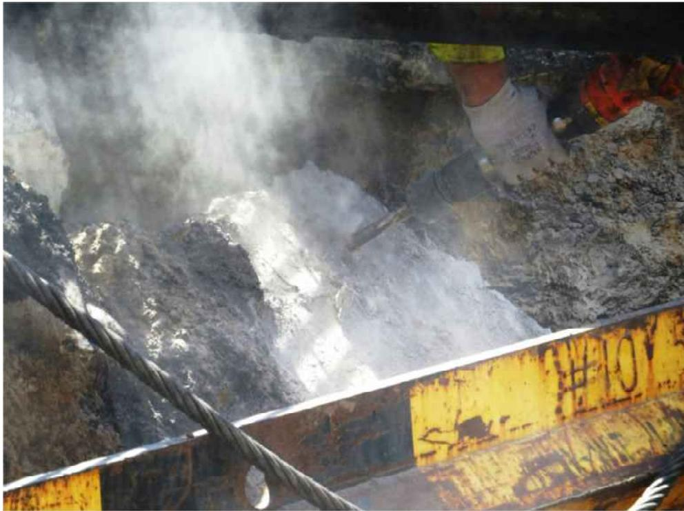
**Figure 11: Concrete Slab Jackhammered to Expose Rebar**
