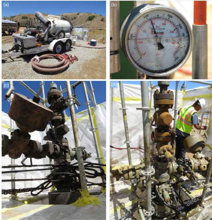
Figure 51: Hydroblasting of SS-25
