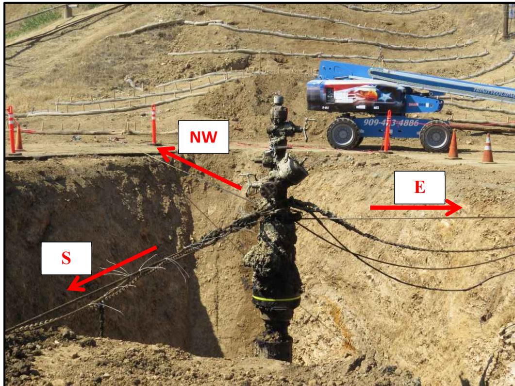
Figure 38: Tensioned Lines for Plumbing the Wellhead
