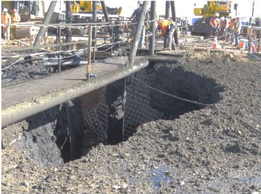
**Figure 9: Net Support Unrolled from Header Bar, Support Lines Tightened to Header Bar**
