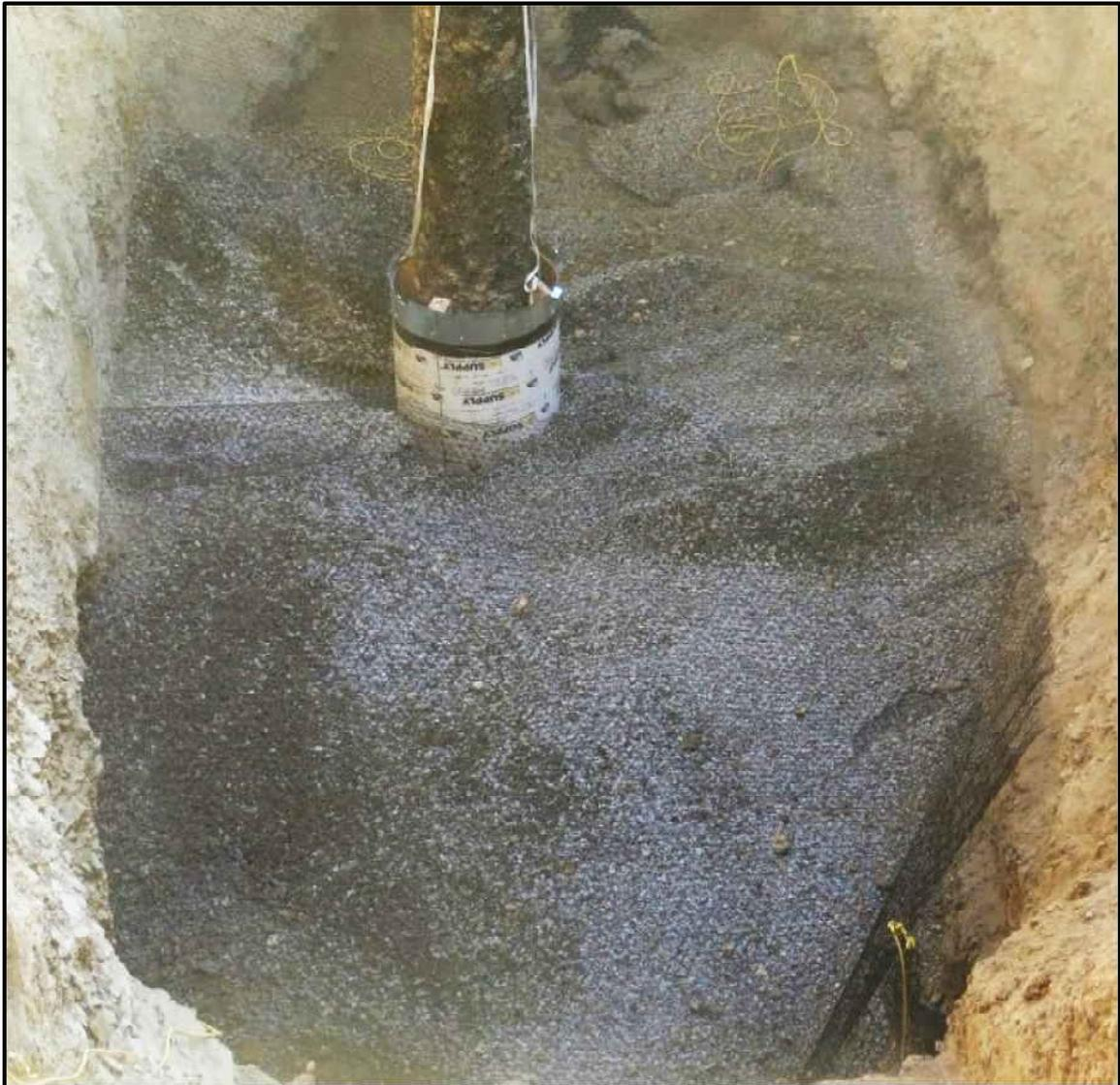
Figure 47: Top of Gravel & Geogrid Layers for Crater Bottom Stabilization
