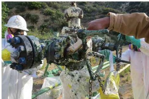
Brass brush used to clean nuts & threads
