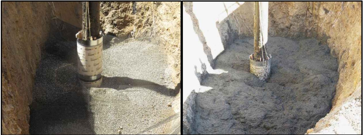
**Figure 51: Crater Before (Left) and After (Right) First Concrete 24 in. Placement, Looking South**
