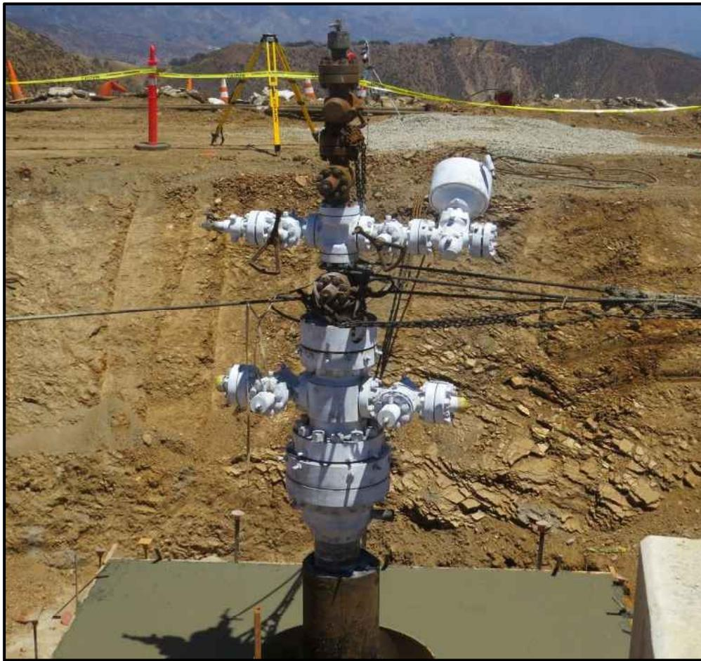
Figure 57: Cleaned Wellhead, Completed Non-Destructive Evaluation
