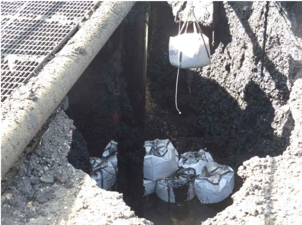
Figure 5: Continued Placement of Super Sack Containers in Crater, South of SS-25 Conductor
