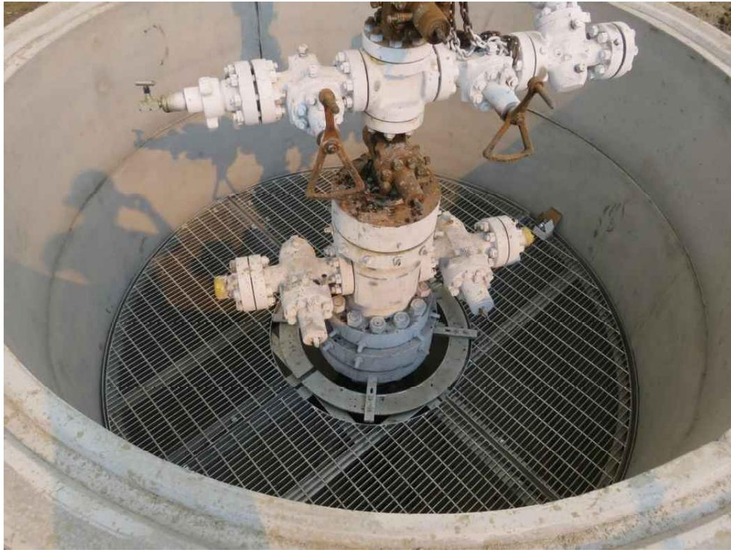
**Figure 61: SS-25's Cellar Fully Installed**
