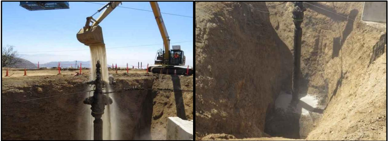
Figure 42: Placement and Mounding of Silica Sand on Crater Bottom
