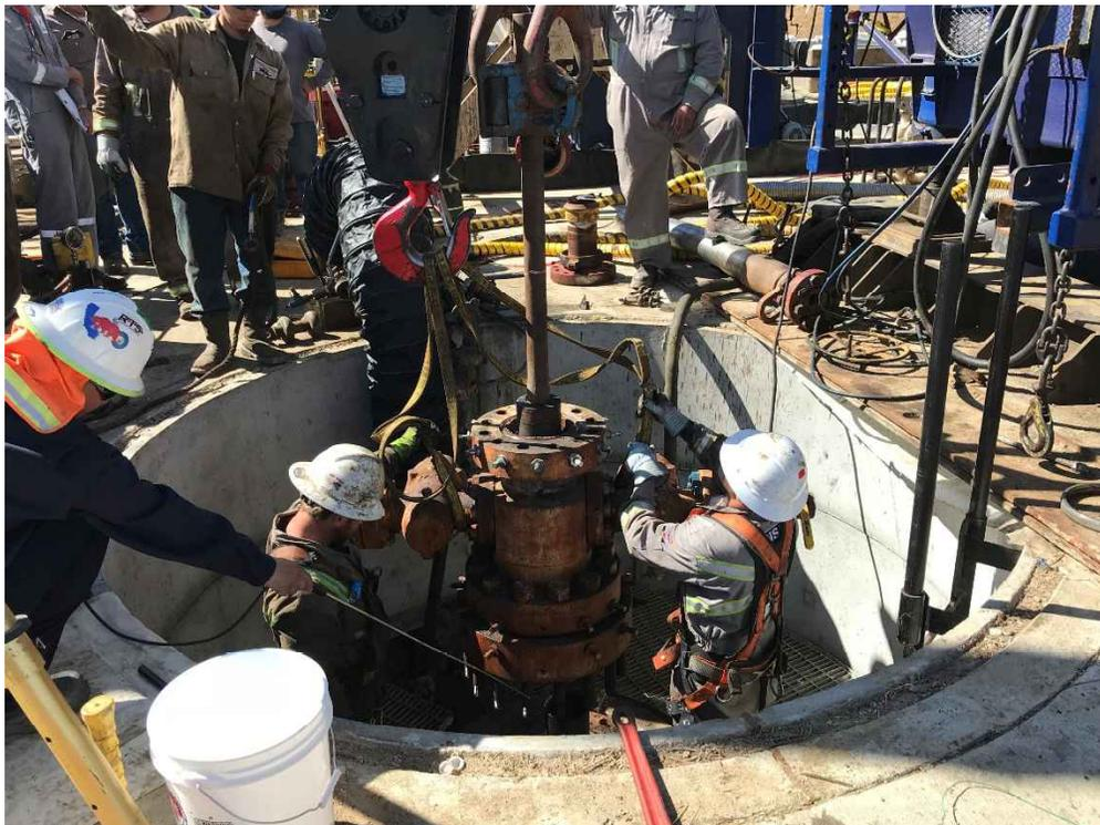
**Figure 16: Removing the SS-25 Tree Assembly**
