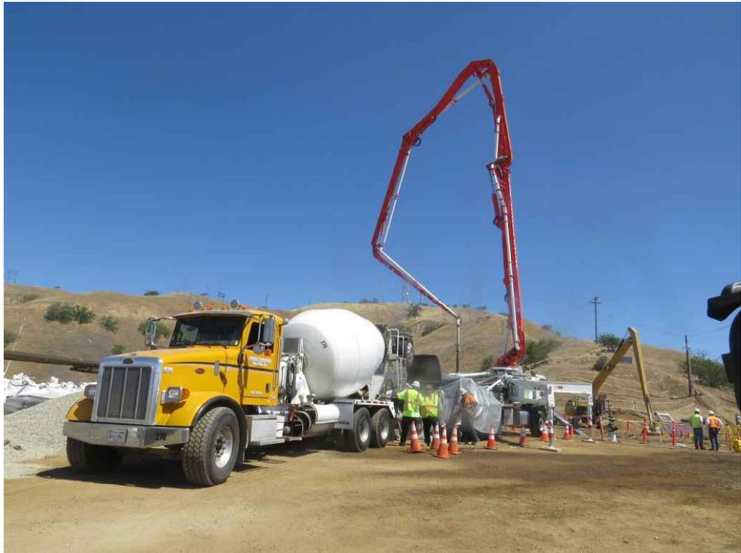
**Figure 49: Concrete Truck and Concrete Pumping Unit on SS-25 Site to Fill Crater**
