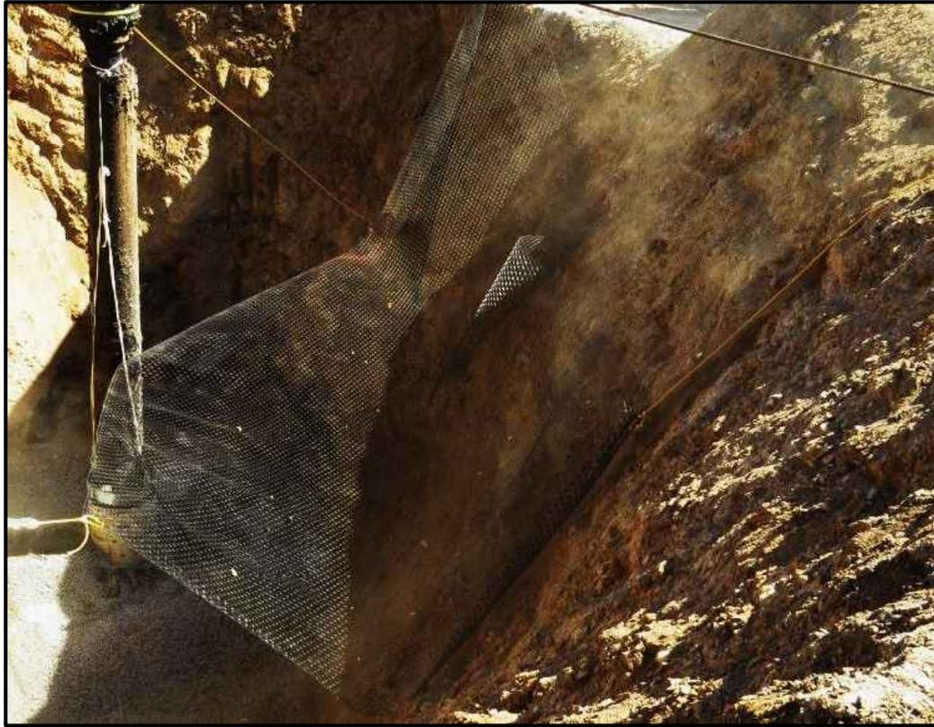
**Figure 46: Geogrid Slid into Crater Bottom with Ropes Tied to Corners and Directed from Surface**
