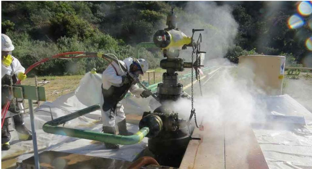
Figure 47: Waterblasting of the Frew 8 Wellhead
