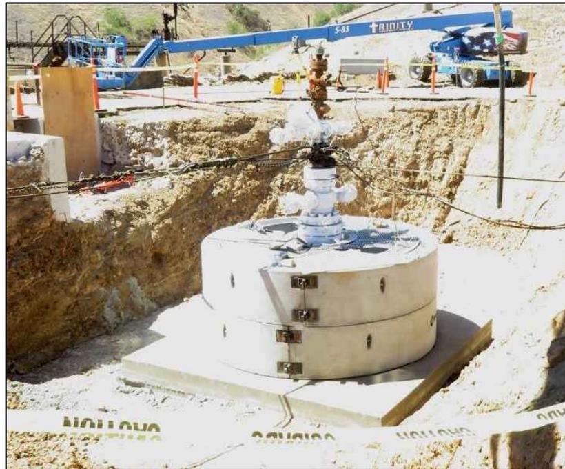
Figure 59: Two of Four 10 ft Diameter SS-25's Cellar Cylinder Segments of 2.5 ft Height Were Installed
