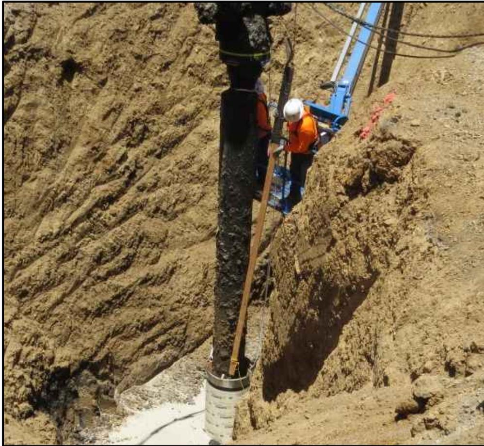
Figure 44: Settling Sonotube Form into Sand and Spacing it Concentric to Conductor
