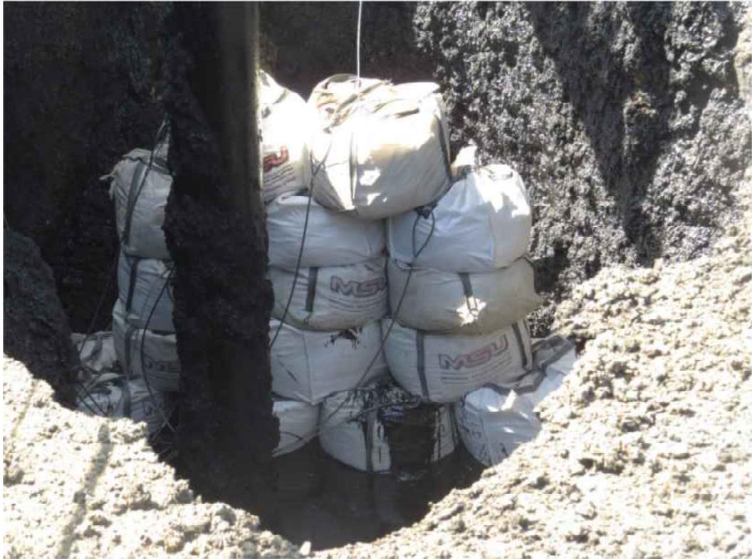
**Figure 6: Complete Placement of Super Sack Containers, Five Layers Tall**
