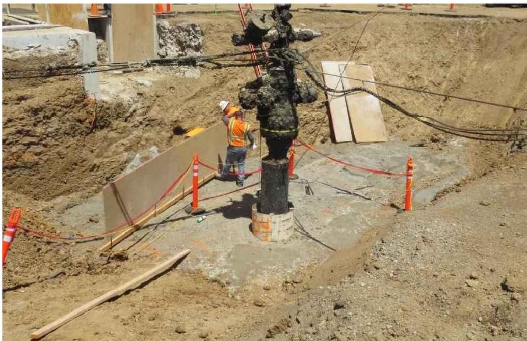
**Figure 55: Construction of Temporary Retaining Walls**
