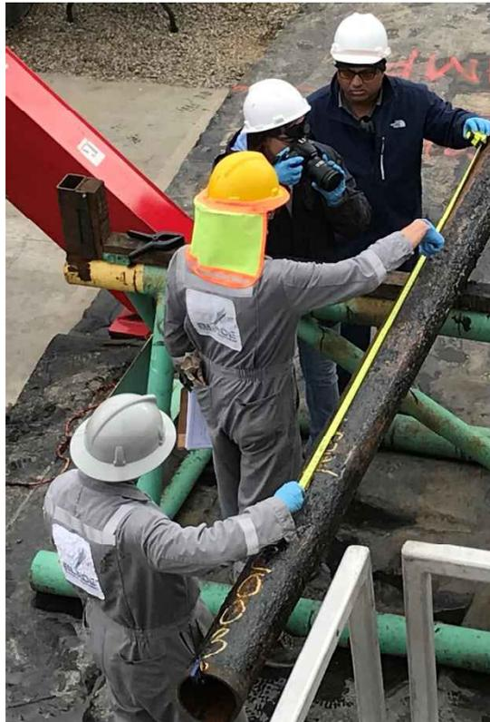
Figure 25: Inspecting a Joint of 7 in. Casing at SS-25
