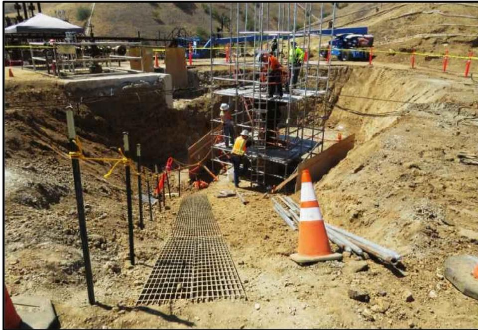
**Figure 56: Egress to Crater and Temporary Retaining Walls Constructed, Looking North**
