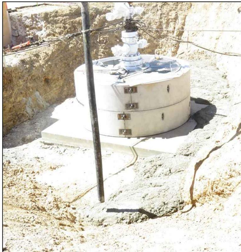
Figure 60: Backfilling Crater with CLSM Slurry Resumes
