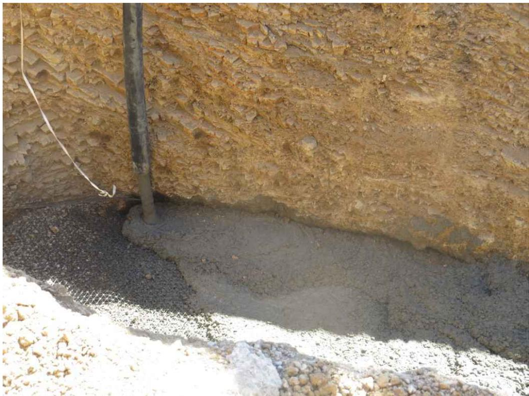
**Figure 50: Begin Placing Concrete in Crater with Pumping Unit**
