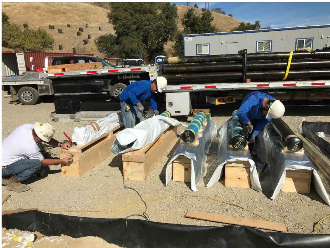
Figure 34: Sealing the Connection Sections in Moisture Barrier Bags Prior to Crating at PS-20
