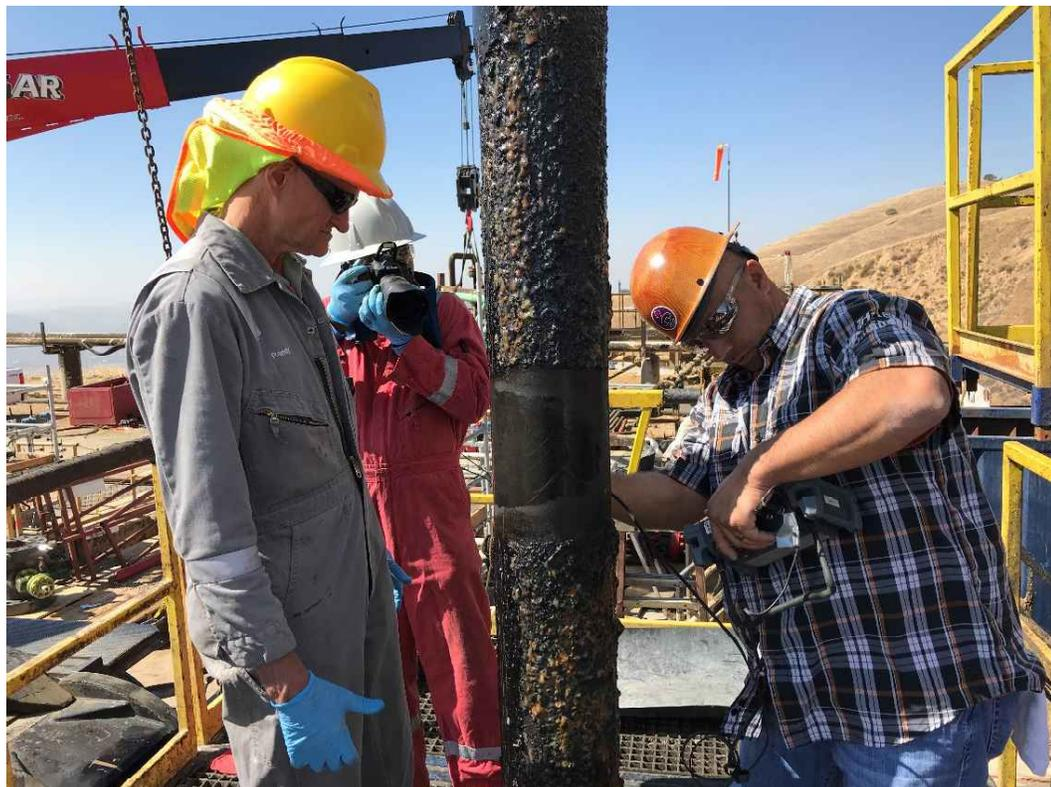
Figure 22: Inspecting the Area Below a Connection Before Cutting the 7 in. Casing
