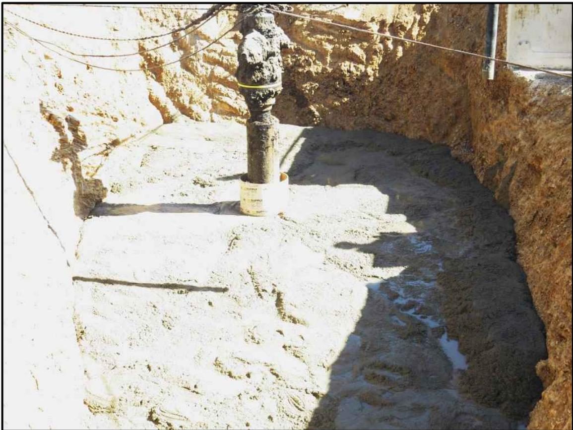
**Figure 52: Crater After CLSM Placement to 12 ft Below Site Grade, Looking South**
