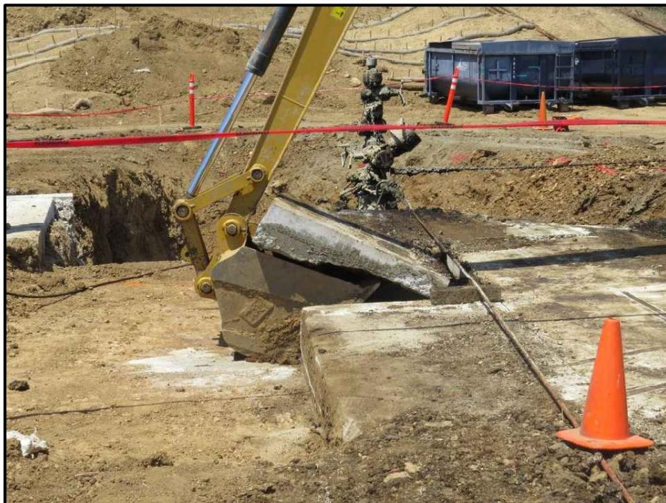
Figure 32: Concrete Well Pad Removed with Excavator
