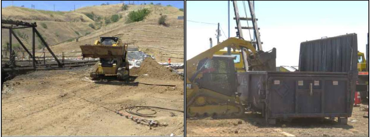
**Figure 17: Excavated Crater Soil Placed in Bins with Front Loader**
