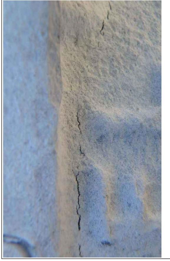
Description : close-up of crack-like within 1st inch
