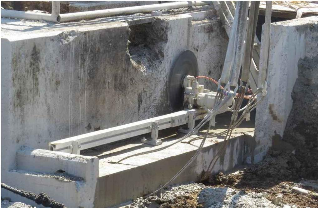
**Figure 27: Insitu Saw-Cutting of SS-25 Pipe Trenches**
