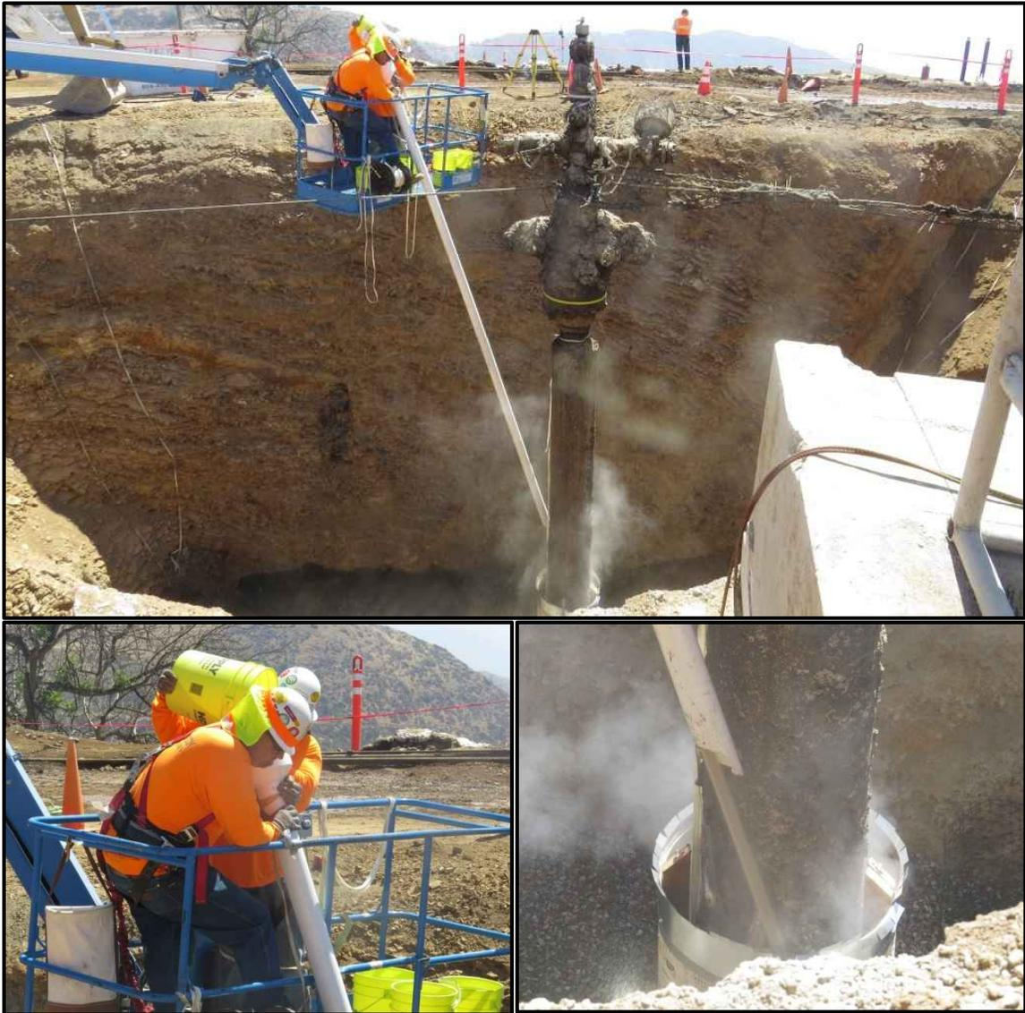
**Figure 48: Filling Conductor-to-Sonotube-Form Annulus with Silica Sand Using PVC Pipe Delivery**
