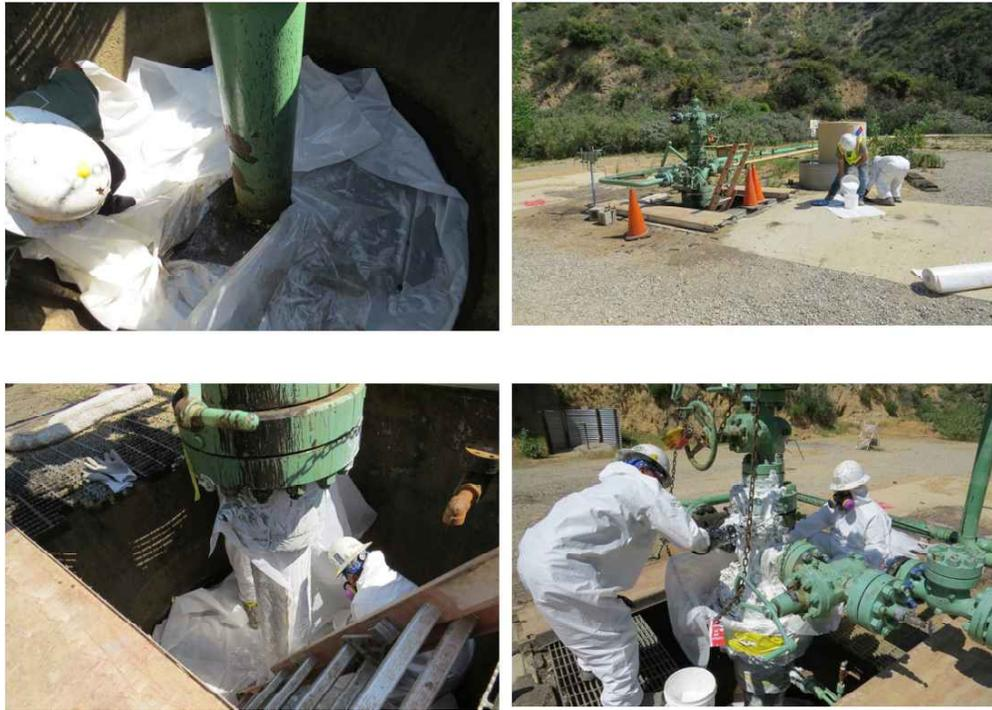
Figure 45: Applying Stripping and Wrapping to Frew 8 Wellhead
