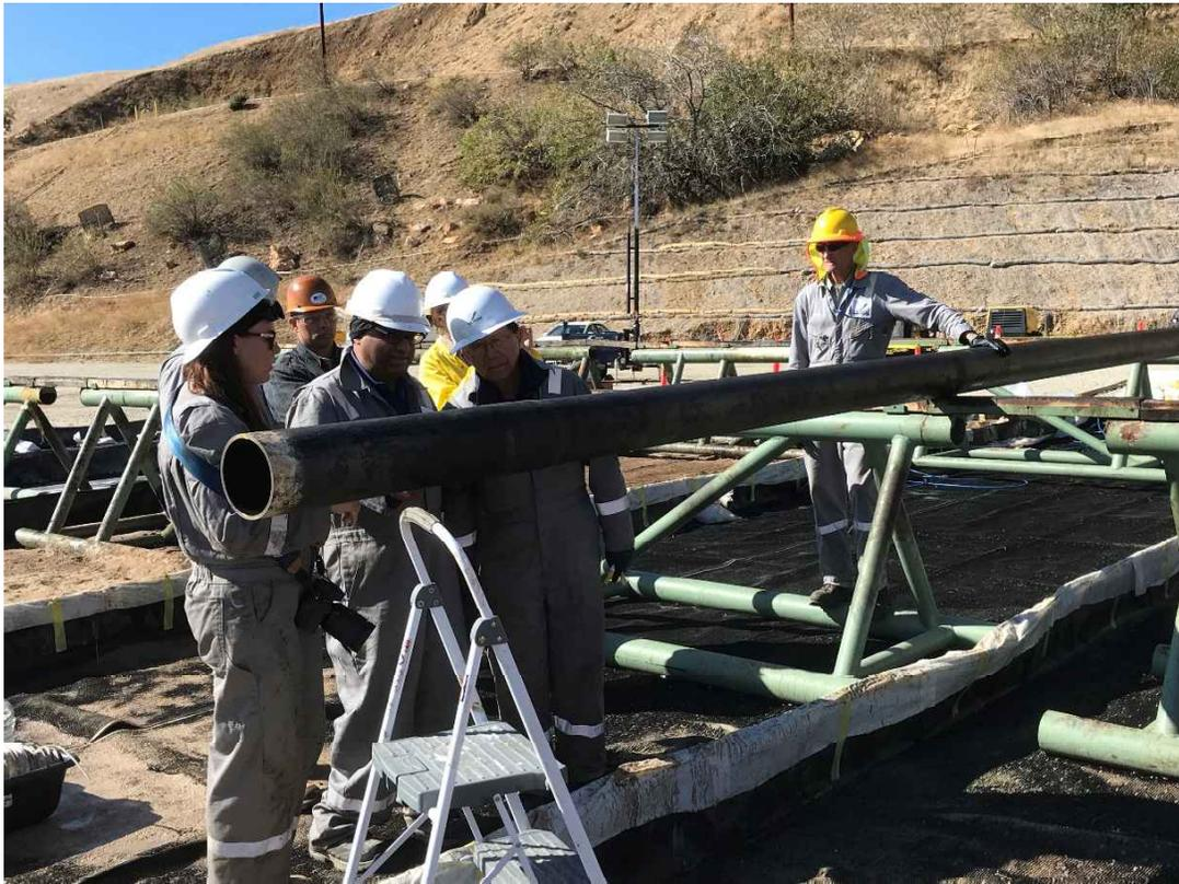
Figure 29: Conducting the Second Inspection of a Cleaned Joint of 7 in. Casing at PS-20
