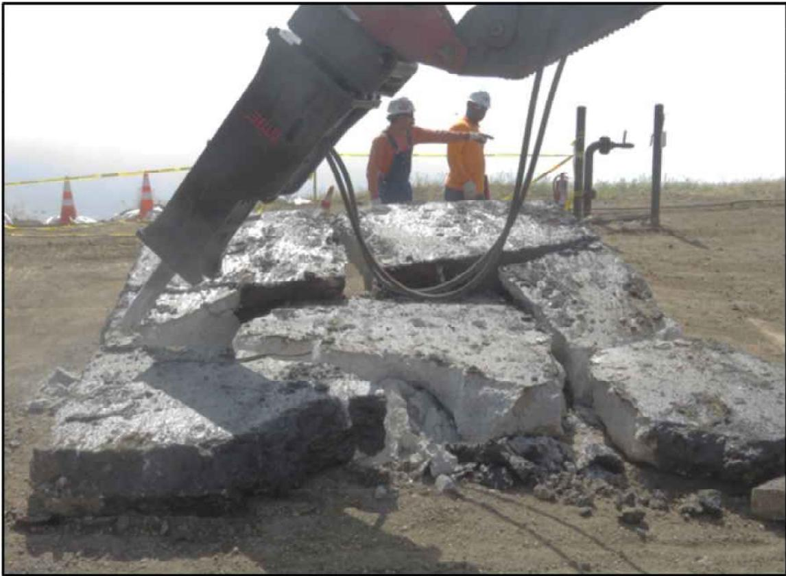
Figure 15: Concrete Slab Jackhammered into Pieces
