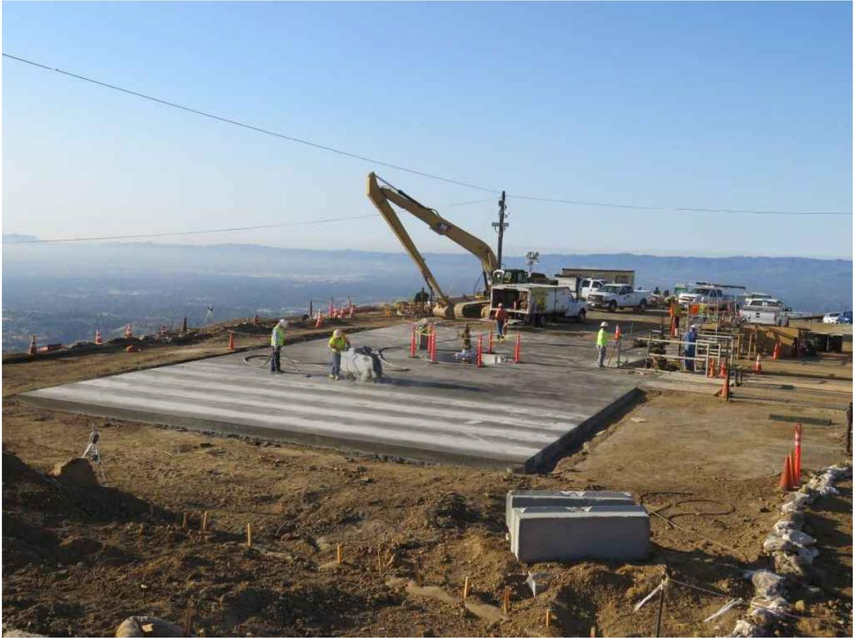
**Figure 63: SS-25's Concrete Mat Installed, Expansion Control Joints Being Cut**
