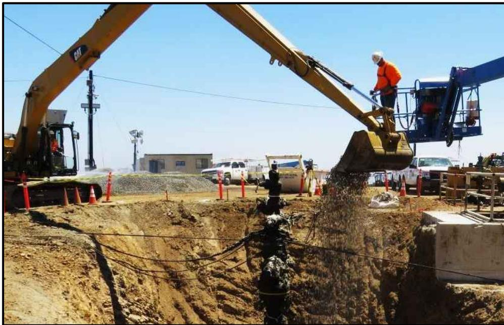
Figure 45: Placement of Gravel into Crater
