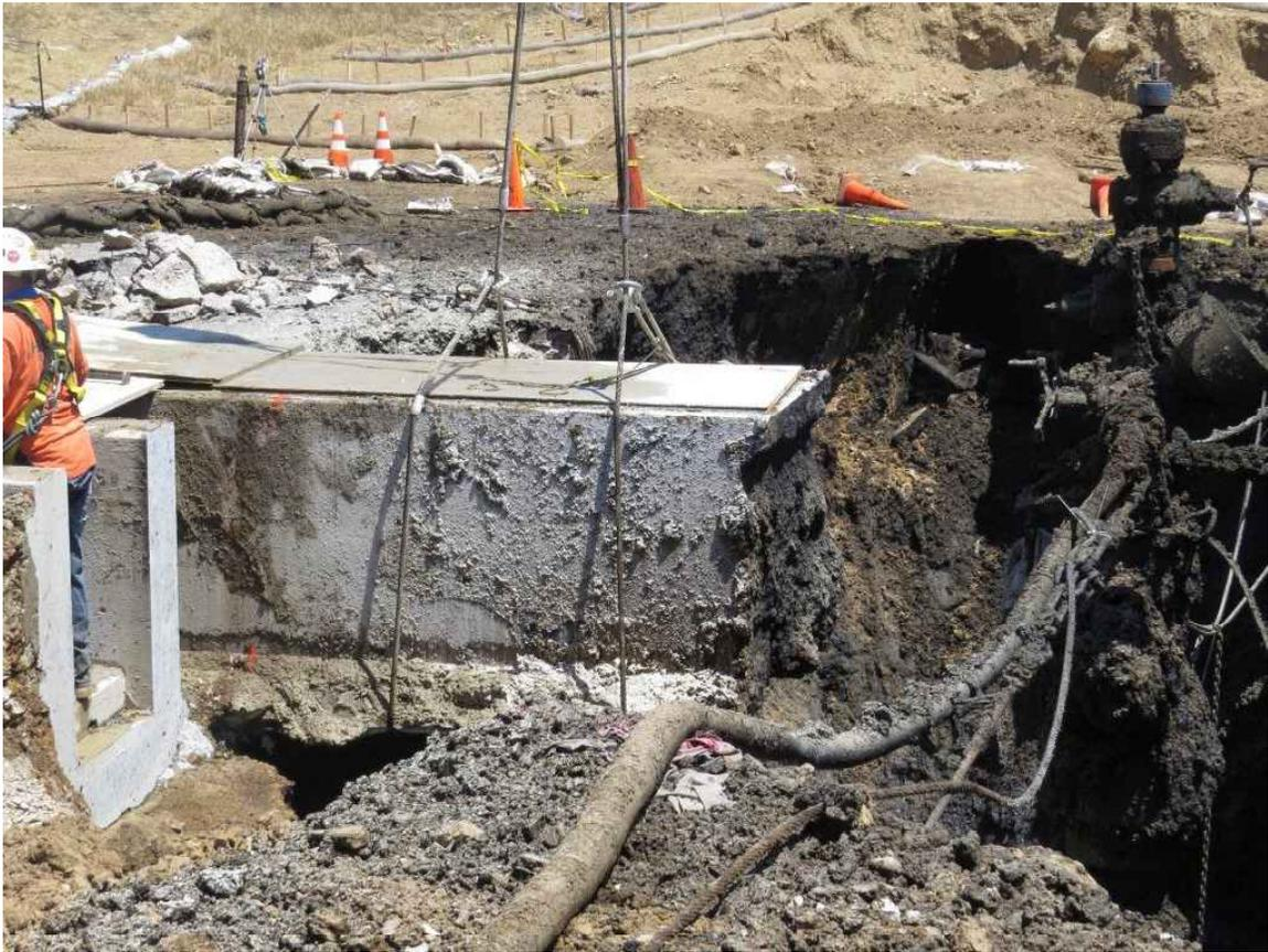
**Figure 26: SS-25 Pipe Trench Segment Affixed to Crane**
