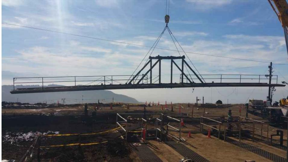
**Figure 19: Wellhead Access Bridge – Crane Lifted from Crater**
