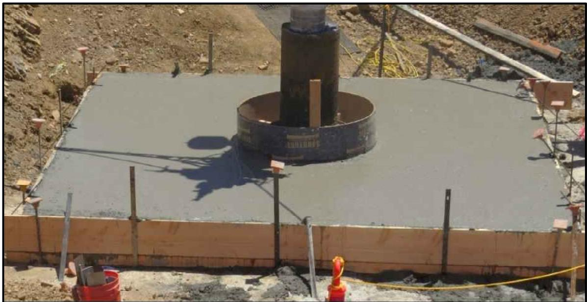
Figure 58: Fiber Reinforced Concrete Mat to Support SS-25's Cellar
