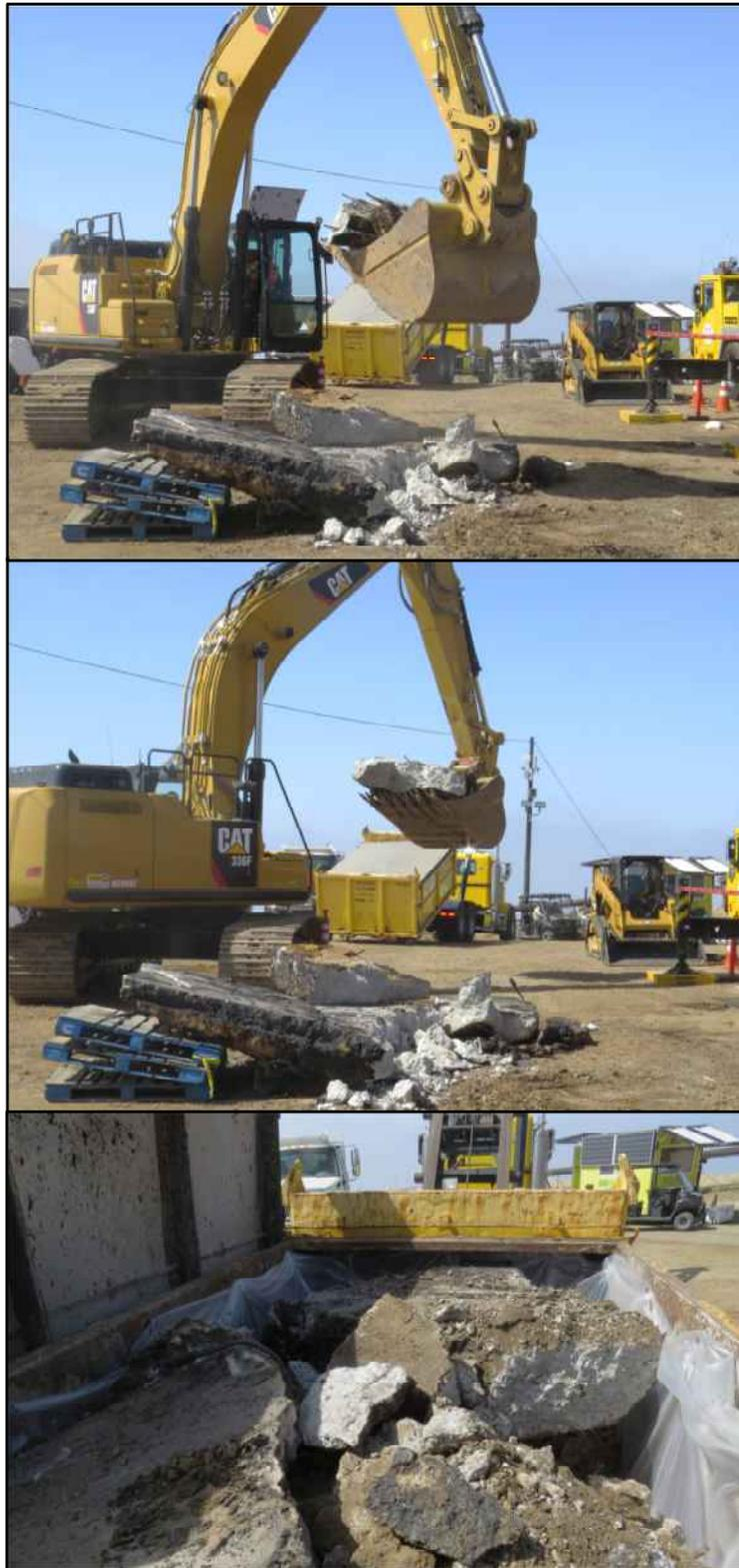
Figure 16: Slab Placed in Bins with Excavator
