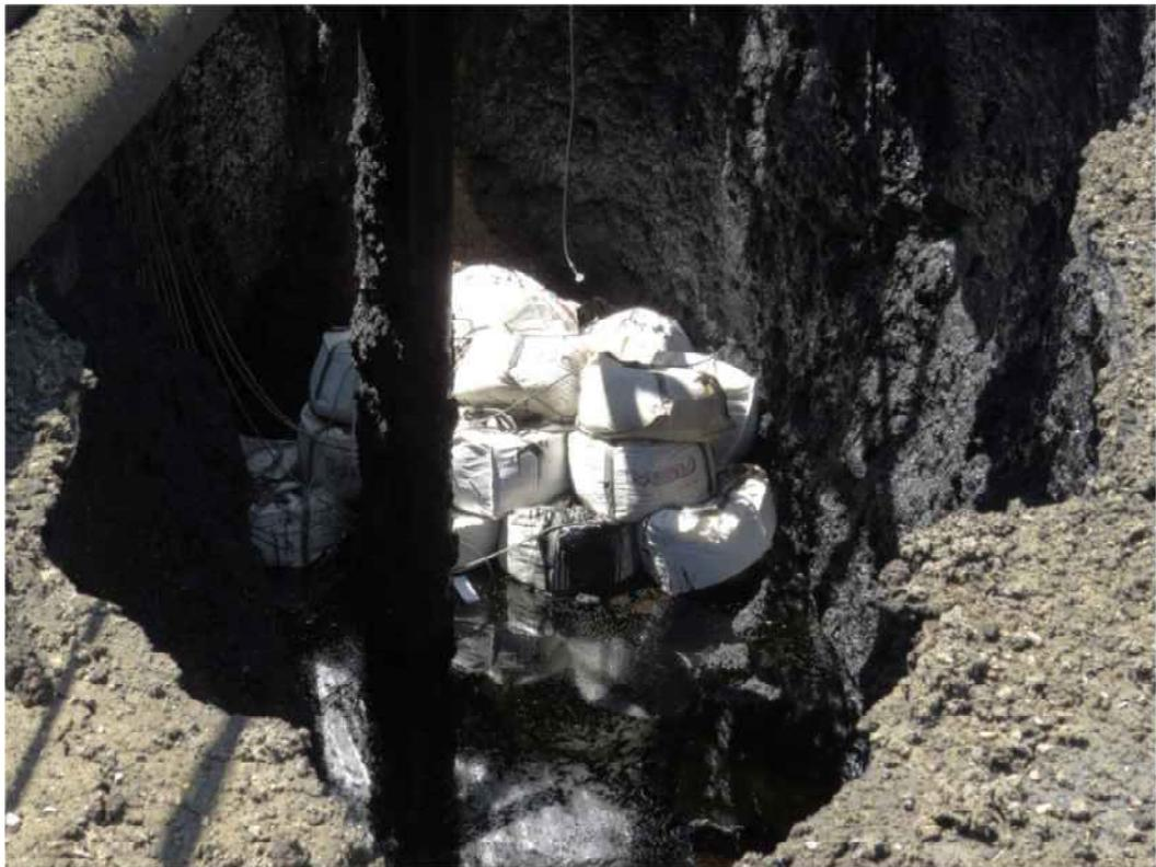
**Figure 7: Super Sack Containers Toppled Overnight; Three-Layers Remained**
