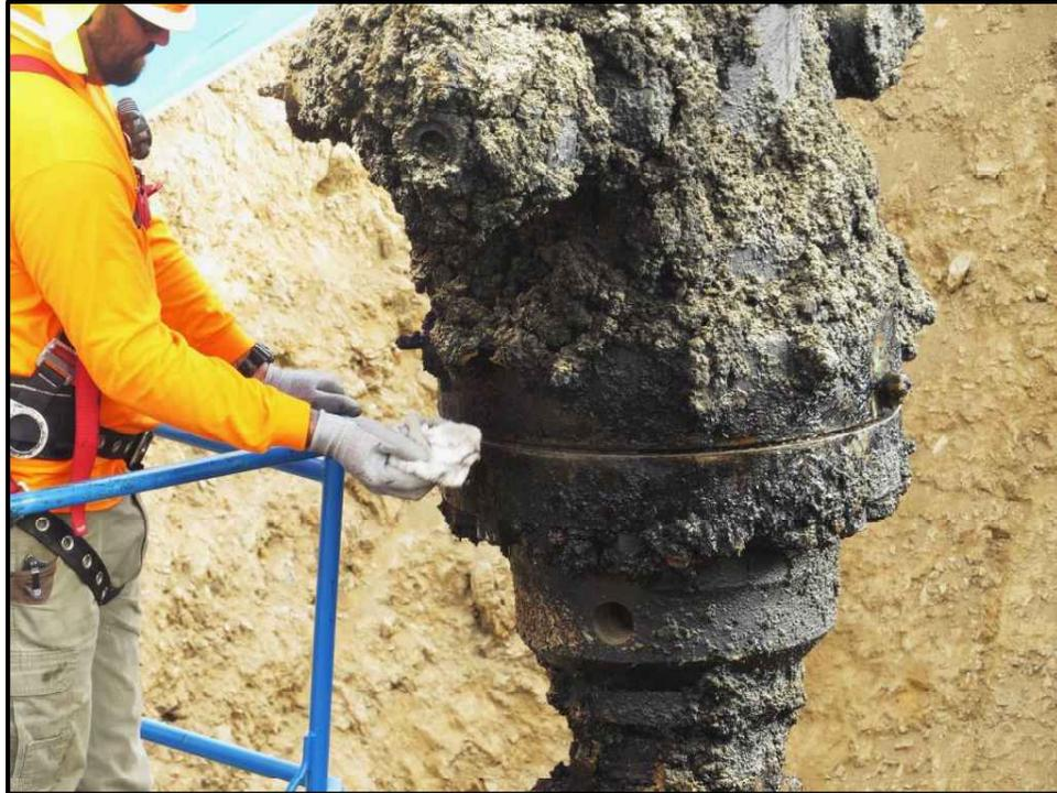
Figure 39: Cleaning the Top Bevel of Bradenhead for Surveyor Sighting Surface
