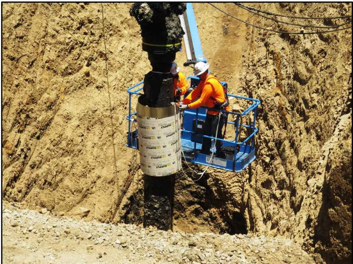
Figure 43: Installation of Sonotube Form around Conductor
