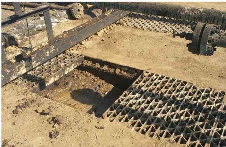
Figure 23: Debris in Pipe Trenches at Site Grade Elevation – Seen Upon Removal of Grating
