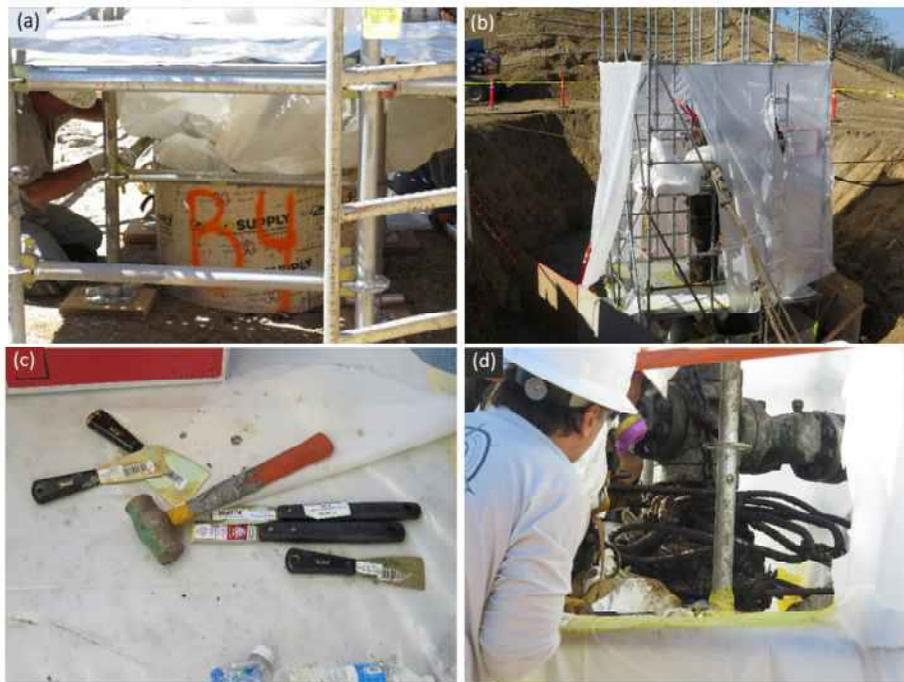
Figure 50: SS-25 Chemical Cleaning and Containment
