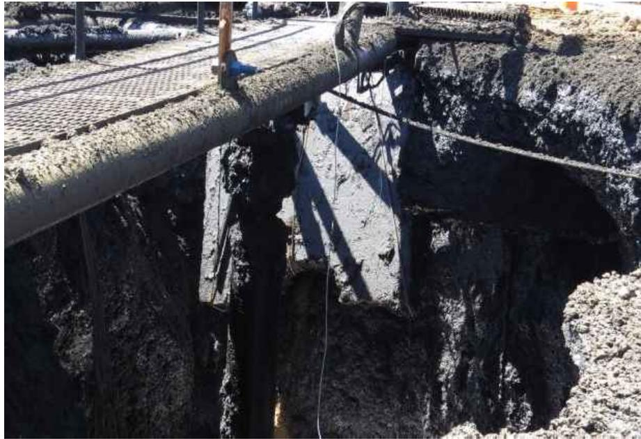
Figure 2: Concrete Slab Suspended from South Edge of Crater
