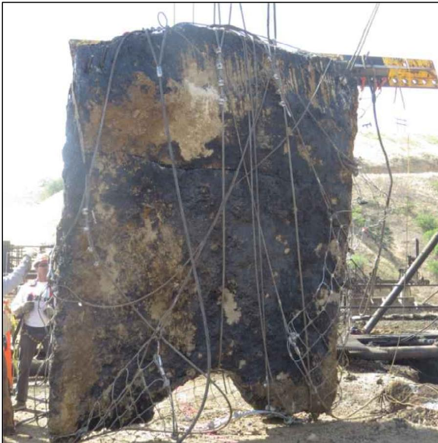
**Figure 14: Safety Straps and Net Support Wrapped Around Slab; View of Bottom of Slab**
