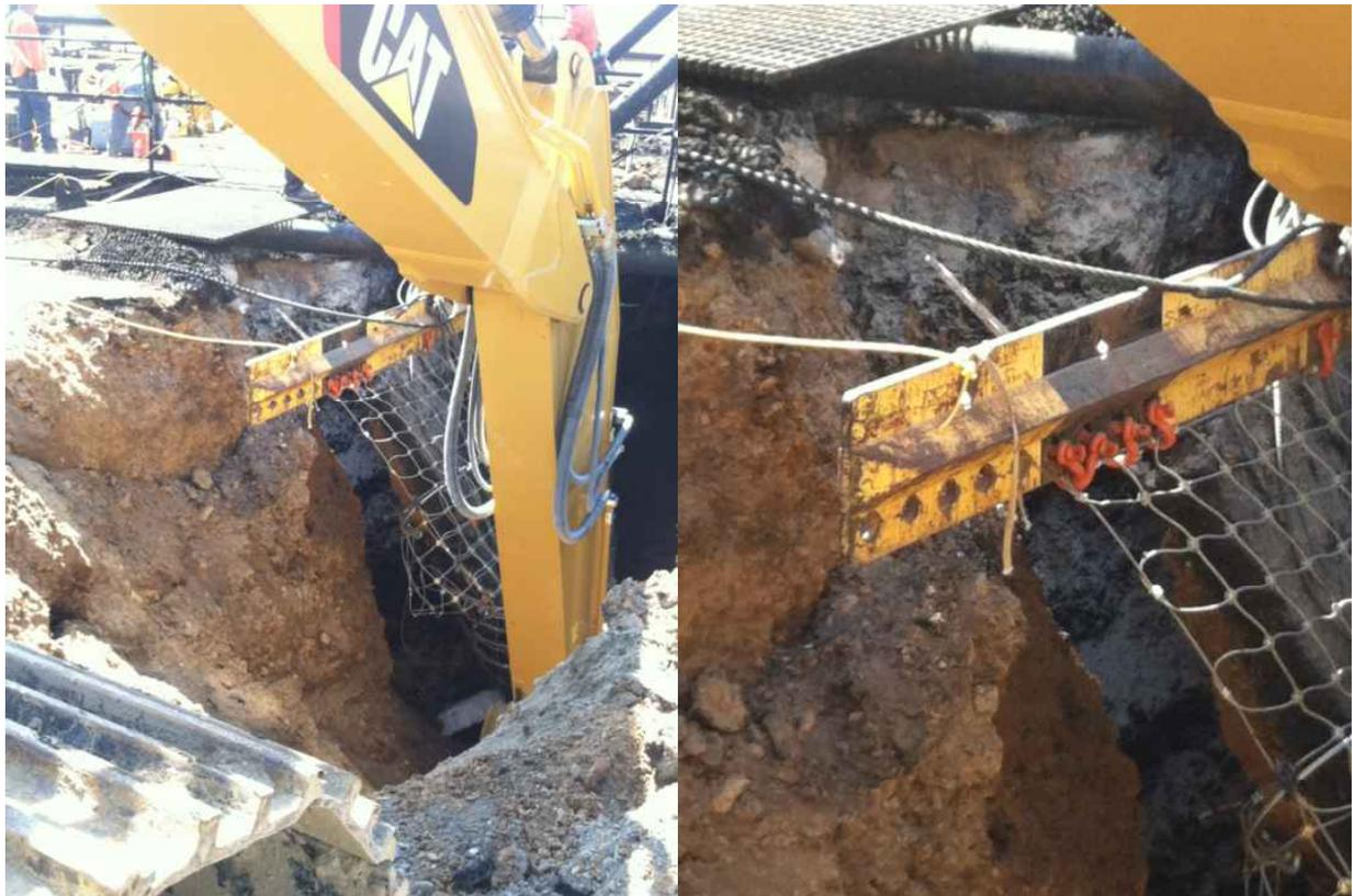
**Figure 12: Reinforcing Bars are Cut (Weight of Slab Supported by Crane)**
