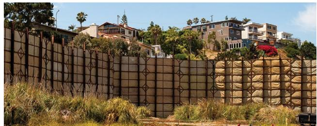
Temporary sound walls, like the ones at PDR, are commonly used in the natural gas industry to effectively block noise from propagating into the surrounding environment.
